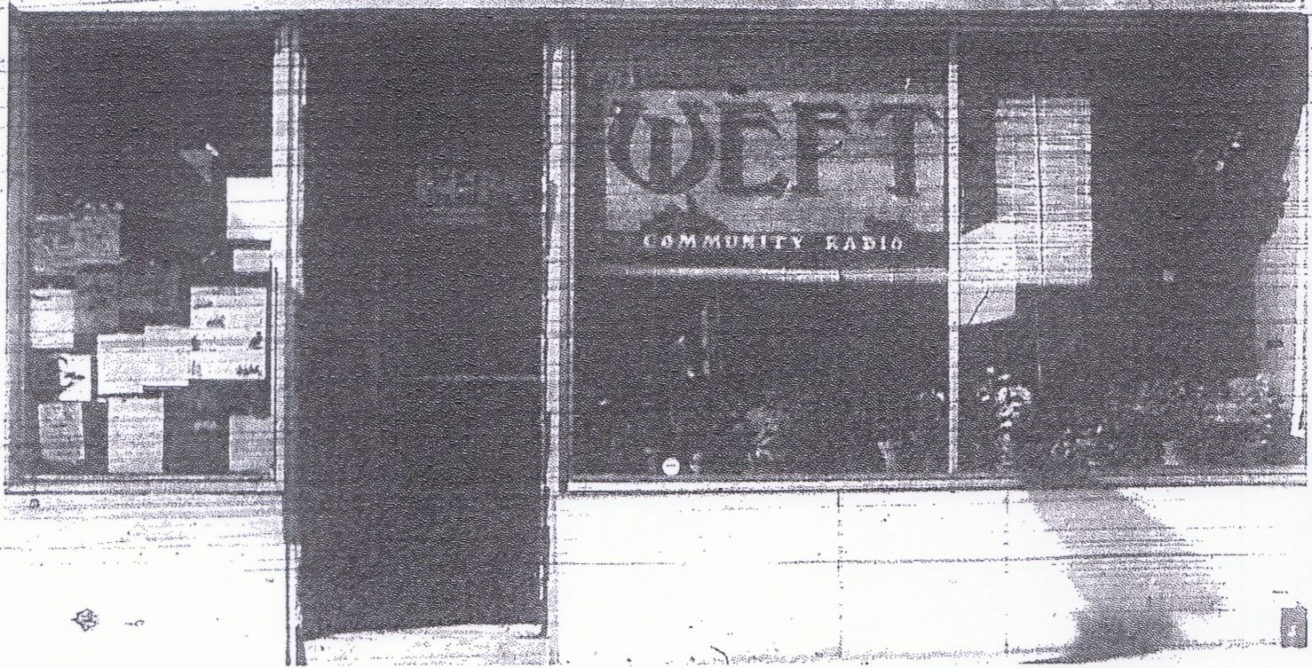
WEFT station office, located at 113 N. Market St., C.
