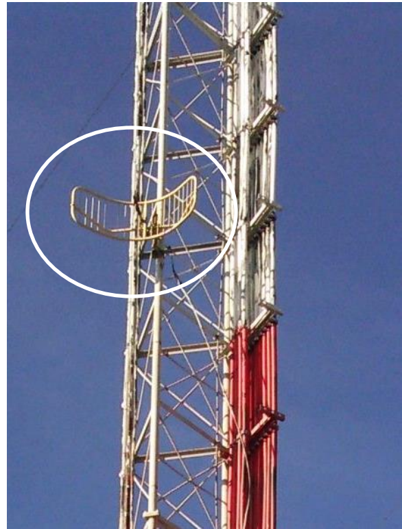
Photo by Lori Serb shows the station to transmitter link (STL) receiver on WEFT's broadcast tower, a gold parabolic grid antenna.
